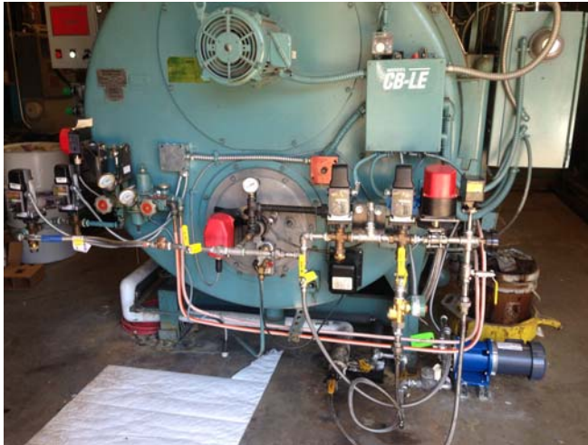
The Dual-Fuel Burner that can Burn both RFO and #4 Oil
